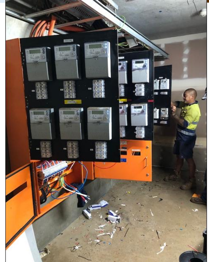
Bldg 2-3 meter repairs
