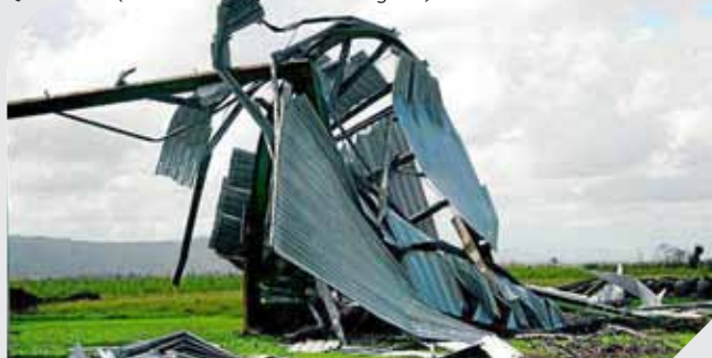
Severe Tropical Cyclone Yasi destroyed farm infrastructure in North Queensland (Source: North Queensland Register).
