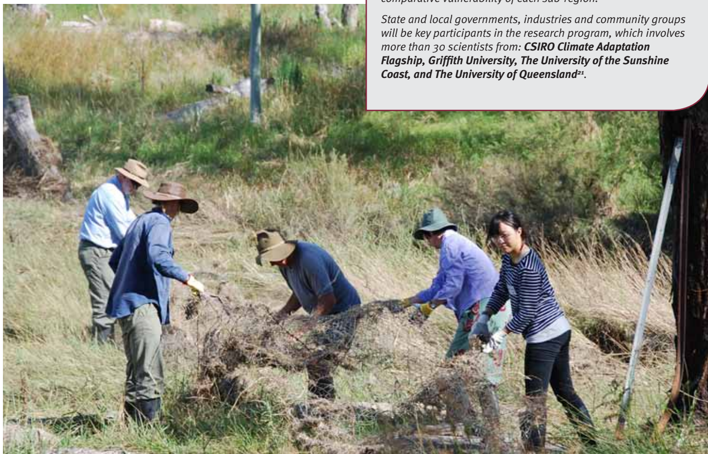
Repairing damaged fencing (Source: www.emergencyvolunteering.com.au )
