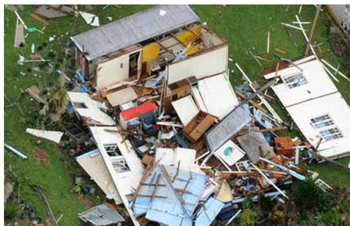
Severe Tropical Cyclone Yasi devastates homes in Tully, North Queensland (Source: AAP).
