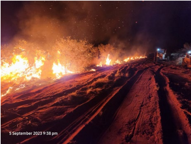
Figure 25. Grader constructing a firebreak to use as a containment line. Image: Bushfires NT
